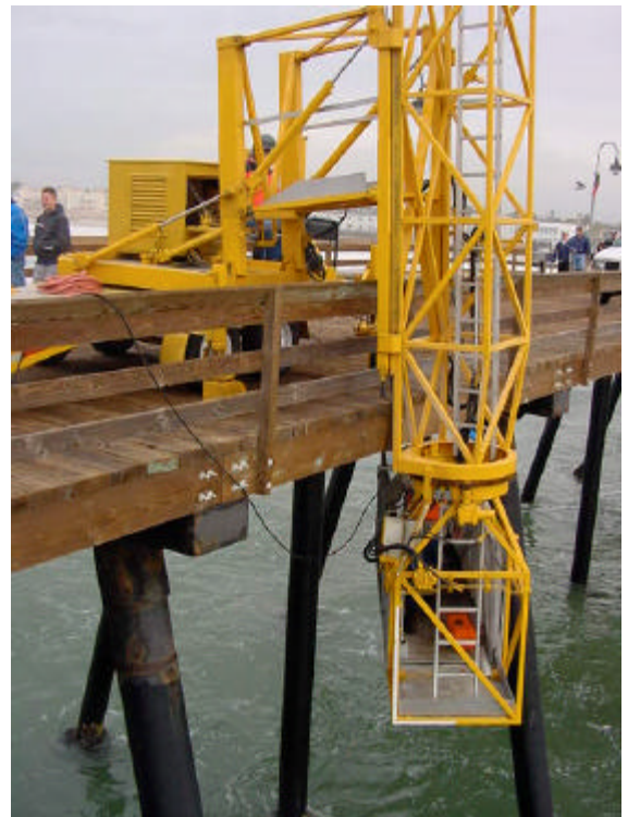
Figure 2. Scripps staff from the Marine Physical Laboratory installing a signal cable on the underside of the Imperial Beach Pier. This cable will connect an offshore sensor package to the lifeguard tower, allowing real-time access to the data. Also shown is the computer system that was installed in the lower floor of the lifeguard tower. This system forms the hub for the environmental sensors that are located on the pier.
