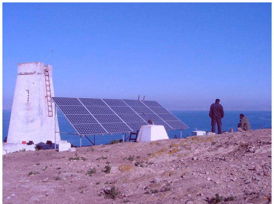
Figure 1. Helicopter transport was used to move the scientific instruments and power system to the Coronado Island. Shown is the solar panel system that powers the CODAR system on the islands. Antennas located on the old lighthouse (antennas not visible) provide the wireless link to Point Loma.
