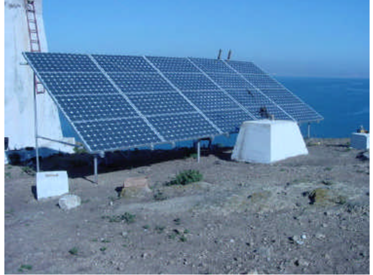
Fig. 14 Solar panels secured to Ground Trac system.
