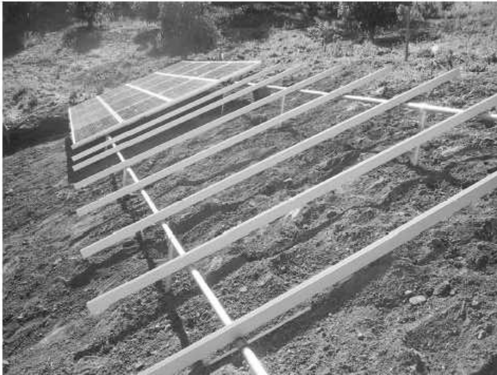
Fig. 12 Ground Trac System by Professional Solar products, showing aluminum support rails, and pipe sub-structure
