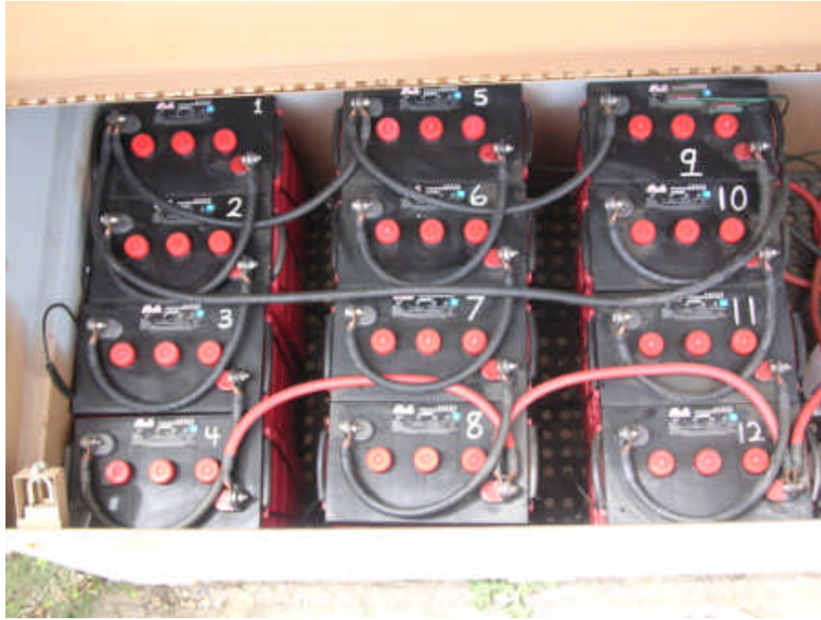
Fig. 2 Battery bank showing series and parallel configurations. 1-4, 5-8, and 9-12 are configured in series, each giving 24 volts DC. These three series are then paralleled.
