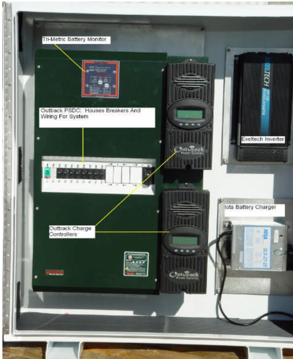
Fig. 22 Inside Enclosure Detailing Various Components
